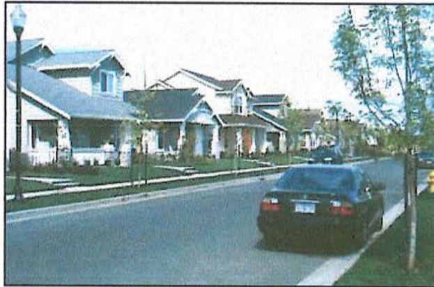
3.2.1.1 a) Homes are sited close to the street with entryways and porches, rather than garages creating an attractive and social environment.
