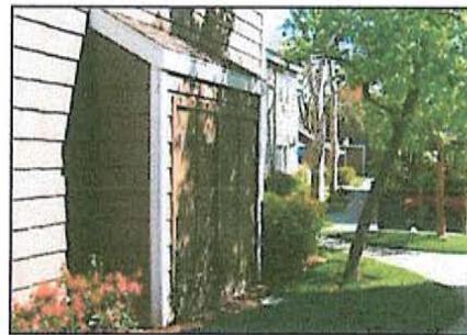
3.2.2.7 c) The screening of utilities can be integrated into the adjacent building through the use of similar materials and architectural elements.
